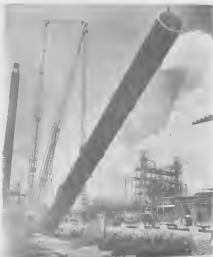
100 TONS of stack supported by towering booms form an interesting geometric pattern against the Caribbean sky.
